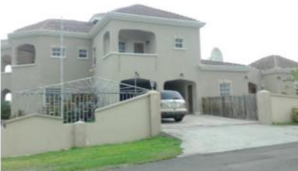
Building from west
