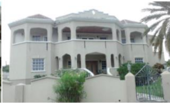
Building from north
