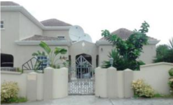
West entrance to house
