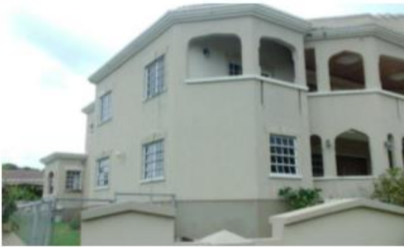
Building from northeast
