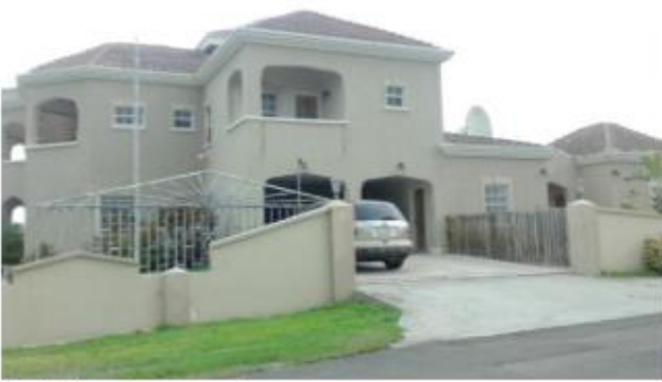
Building from west
