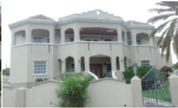
Building from north
